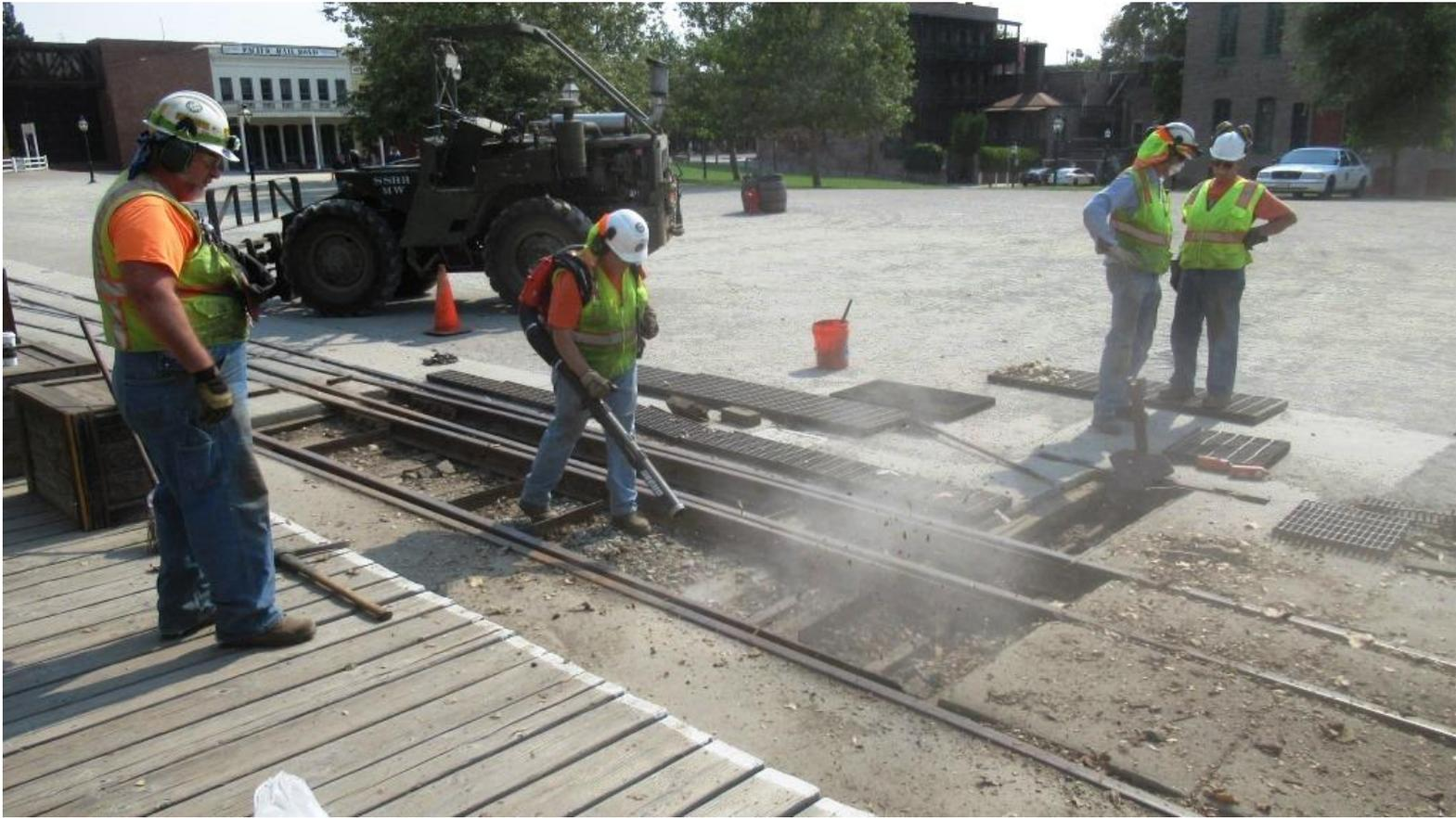
Bill employs the "huff-'n'-puff" machine and utilizes the power of the wind to clean out the switch
