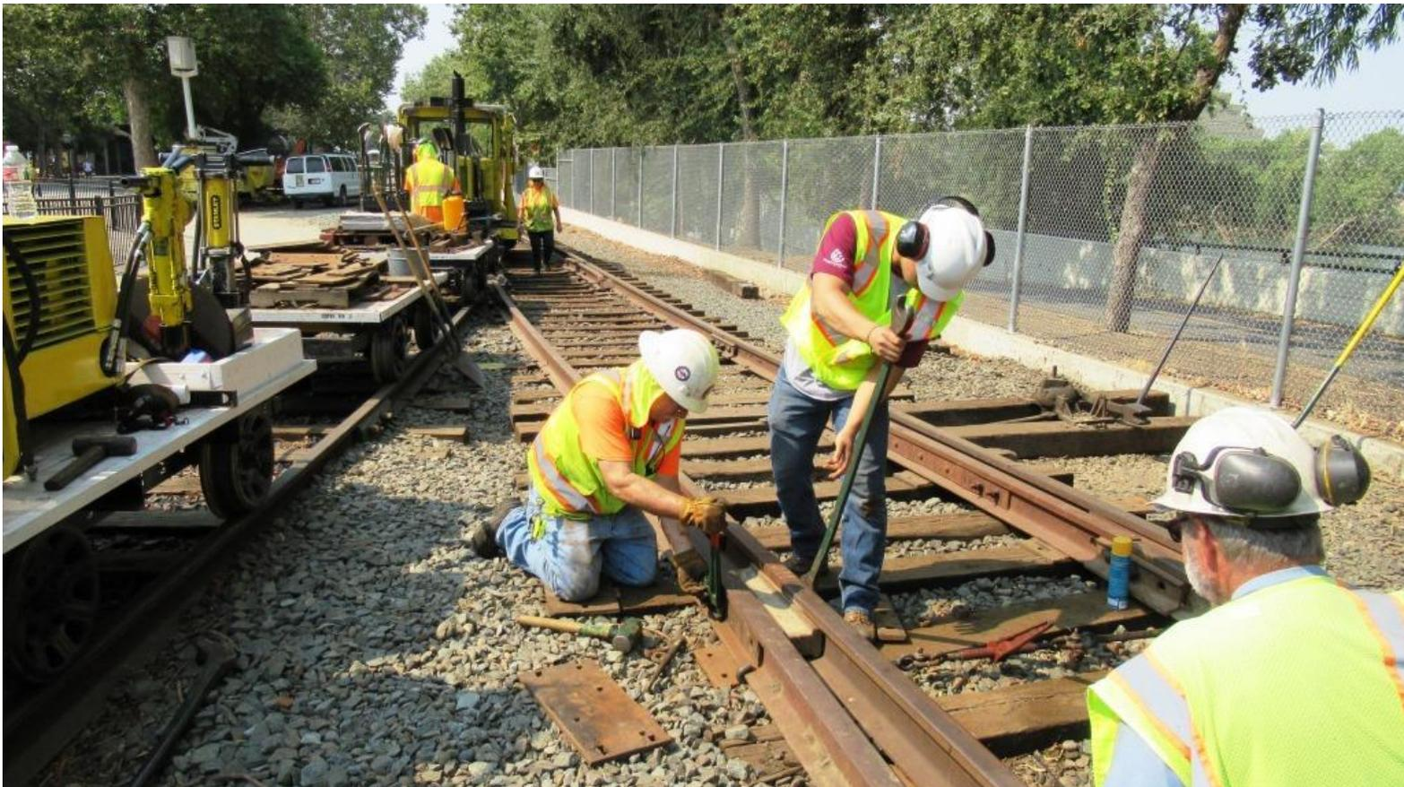
Mike F. uses a monkey-wrench to hold the bolt head as Tavish tightens down the nut on the heel-block
