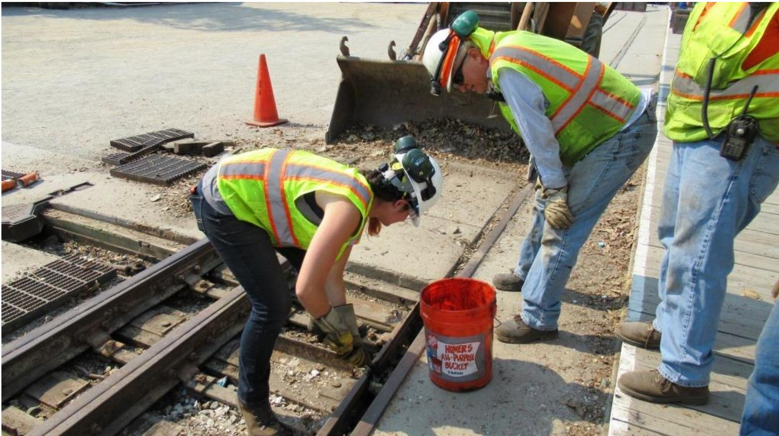
Samantha applies switch-grease to the dual-gauge under Steve's tutelage
