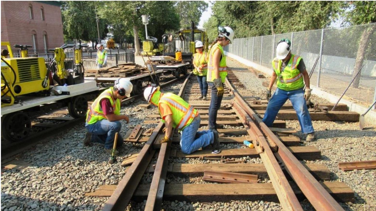
Tavish and Mike H. work on installing the east heel-block while Samantha and Ed adjust the west heel-block
