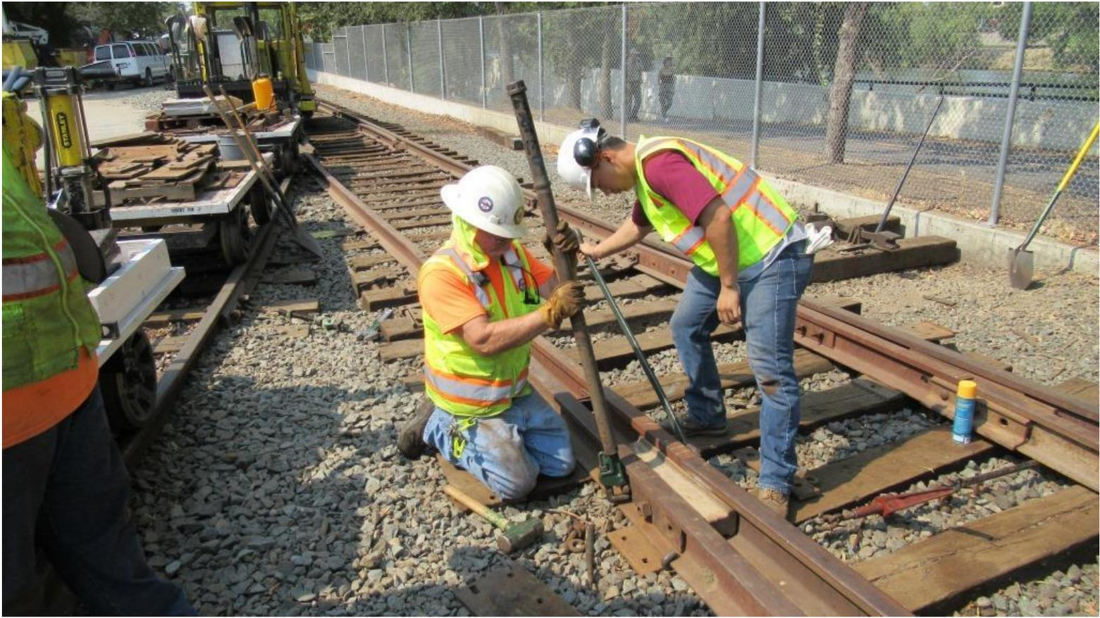
Mike H. uses a “cheater-bar” to provide better leverage on the monkey-wrench as Tavish tightens the nuts on the heel-block
